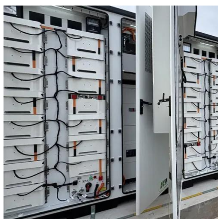
LV-Rack-30KWh Cabinet type battery energy storage cabinet
